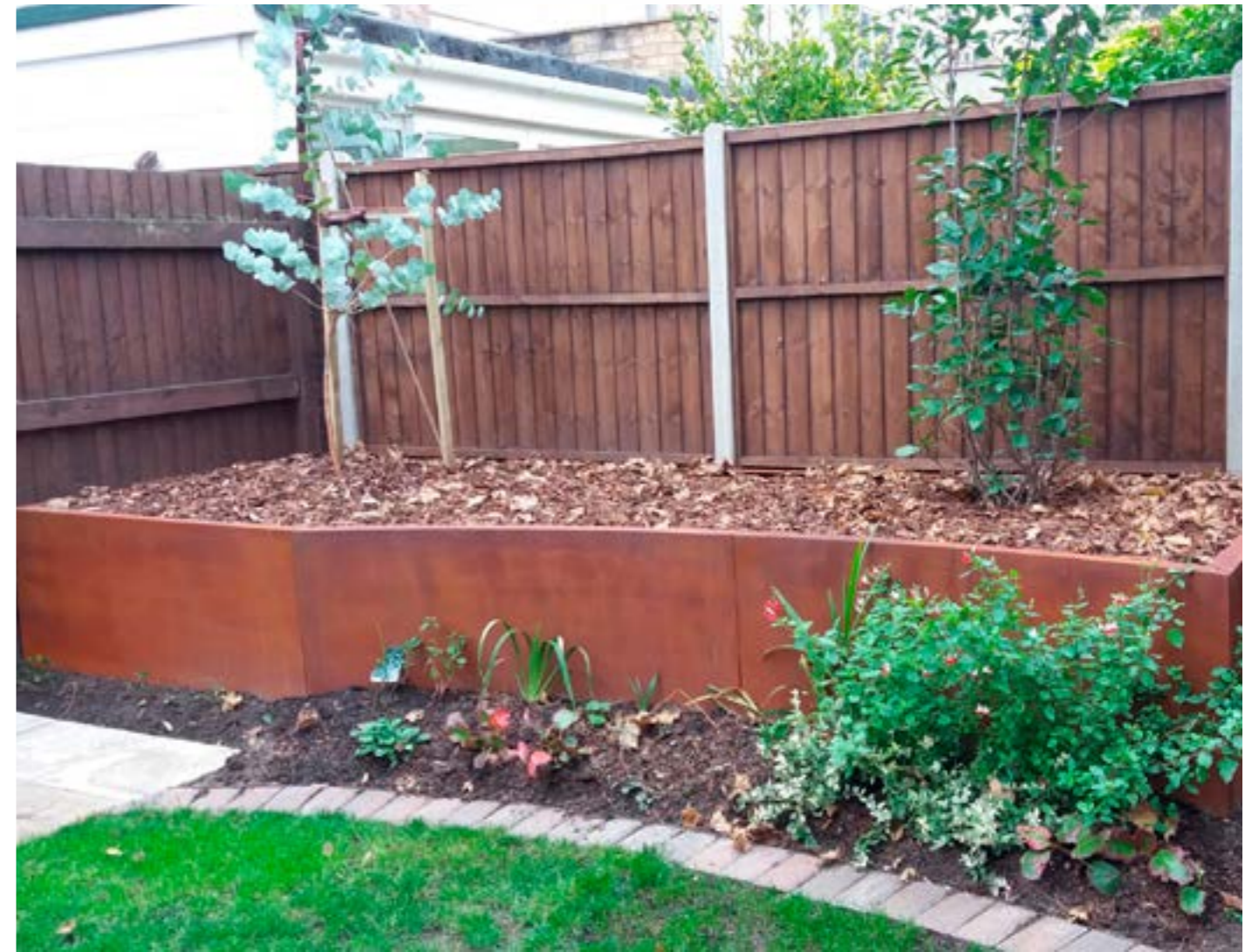
The bed installed on site
